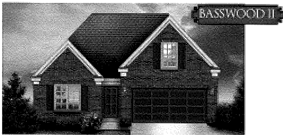
Exterior elevation, with porch and garage.
